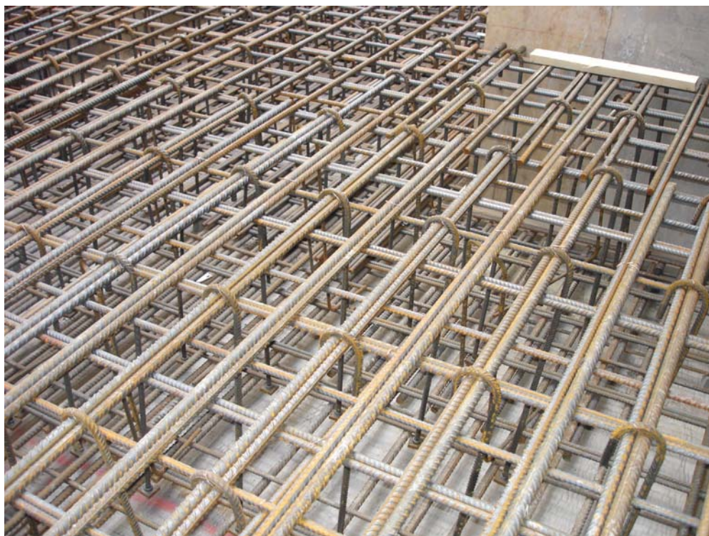
T-headed shear reinforcement in base slab of an approach ramp
