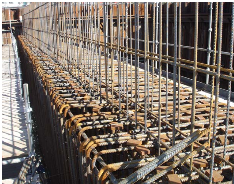
T-headed shear reinforcement \varnothing 32\text{mm} in large beam
