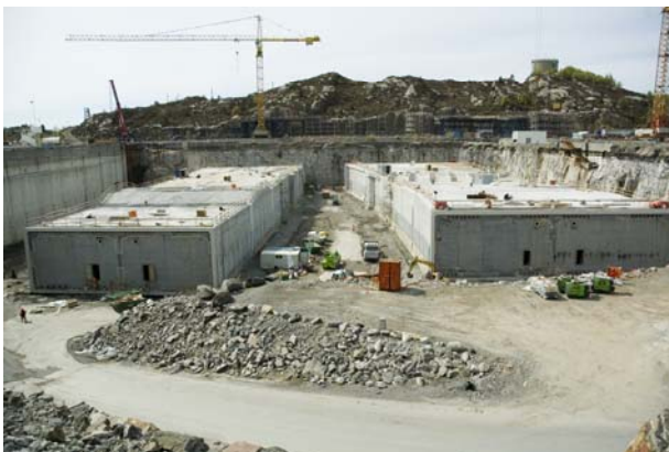
Construction of tunnel elements in dry dock (Picture: Byggindustrien)
