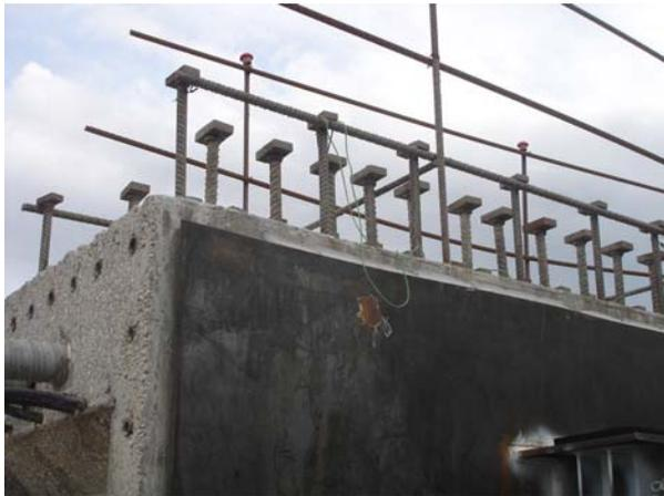
Close-up of top slab beam with protruding T-headed bars
