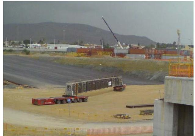
Transport of prefabricated beam
