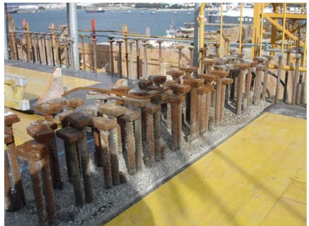
T-headed bars of supporting beam with formwork for top slab in place
