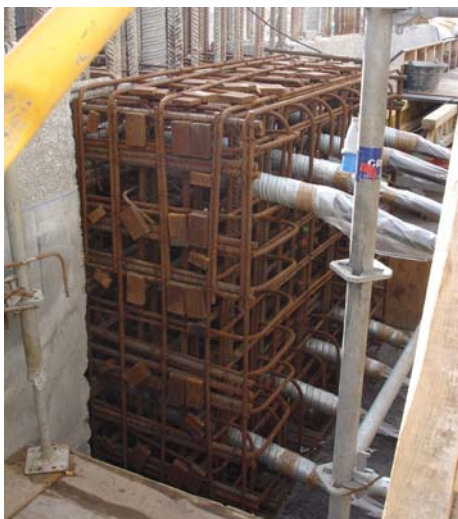
T-headed reinforcement at anchorage of post tensioning cables
