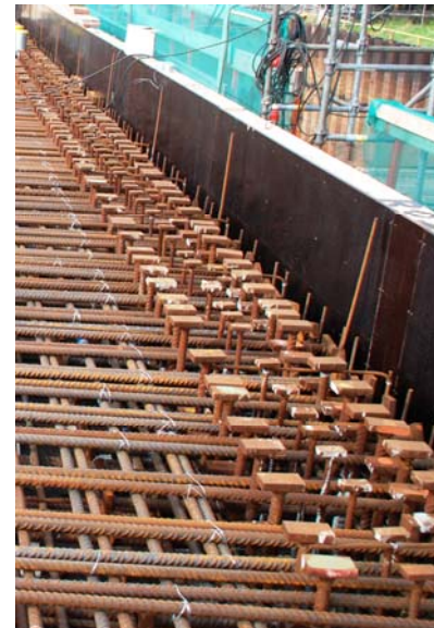
Frame corner with T-headed bars
