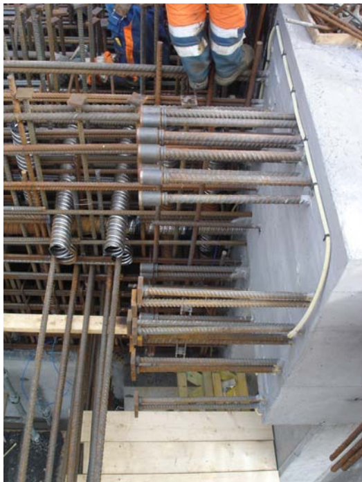
Splicing and anchorage of large diameter rebar
