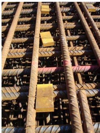
Fixing of T-headed bars by tie wire
