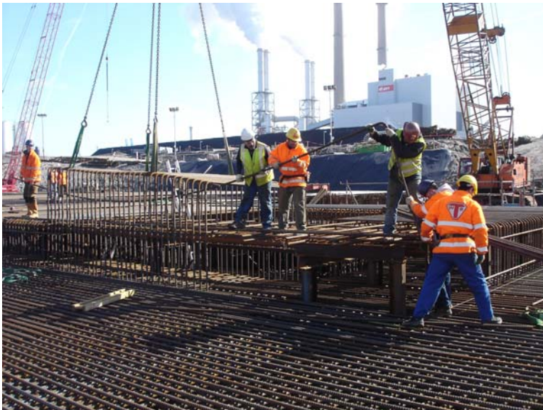
Labor-intensive and inconvenient placing of long bend rebar
