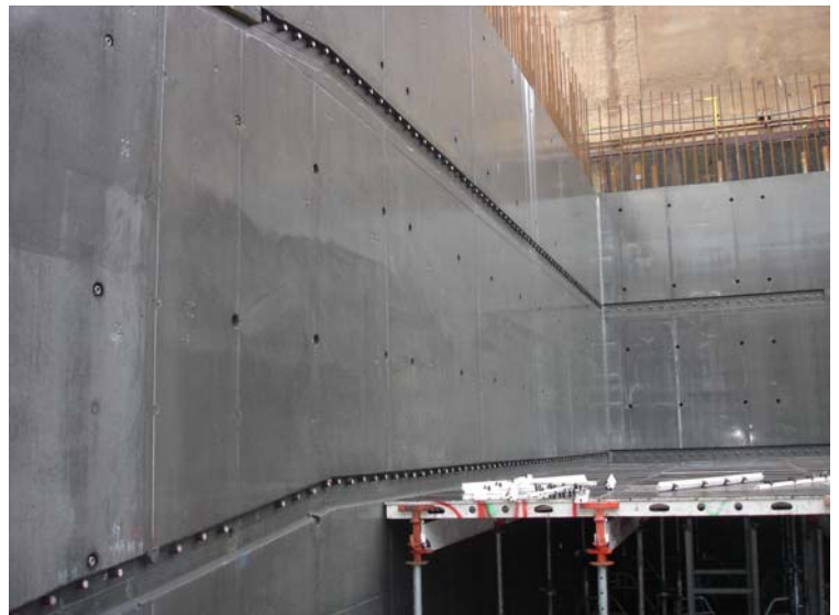
Example for wall-slab-connection using HRC 400
