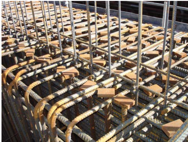
T-headed shear reinforcement Ø32mm in a beam
