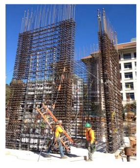
Further is it important for the use of special rebar components, as anchorages and mechanical splices, that these have sufficient capacity. Otherwise the actual ductility of the rebar will not be utilized, creating weak links – even if the rebar itself is strong and ductile.
