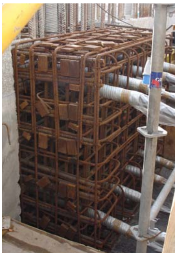
T-headed reinforcement at anchorage of post tensioning cables
