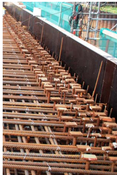
Frame corner with T-headed bars
