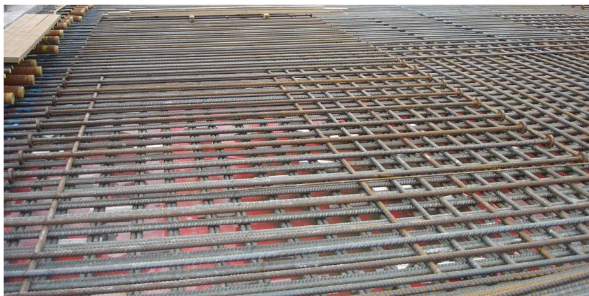
Additional T-headed reinforcement to cover peak bending moments in a slab: no anchorage length
