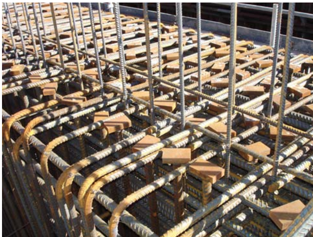
T-headed shear reinforcement Ø32mm in a beam
