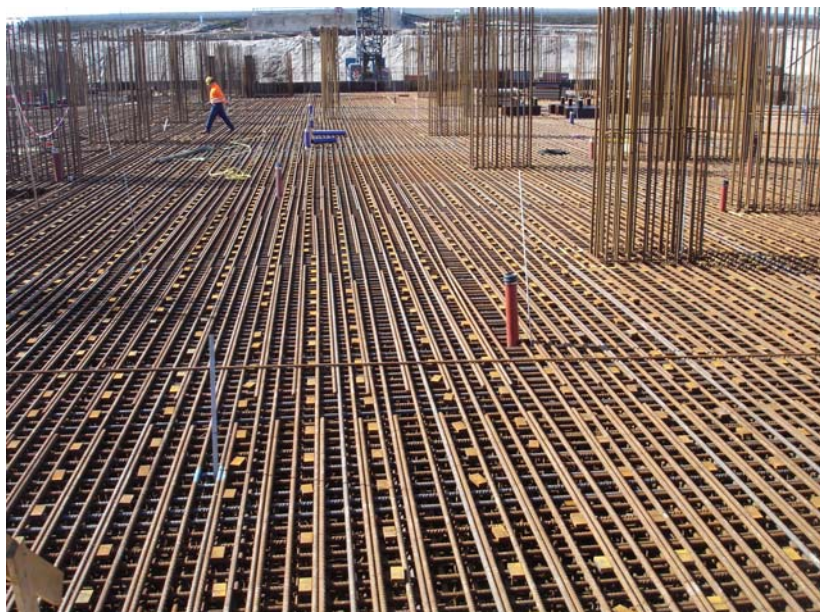
Easy and quick installation of T-headed shear reinforcement in a slab
