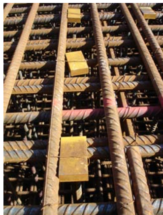
Fixing of T-headed bars by tie wire
