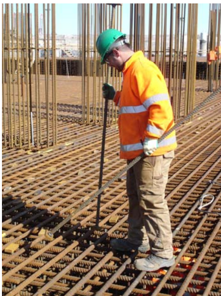
Easy and quick installation of T-headed shear reinforcement in a slab
