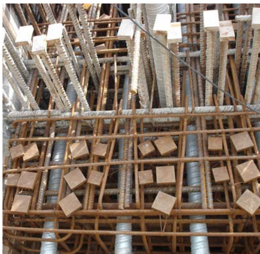
T-headed reinforcement at anchorage of post tensioning cables
